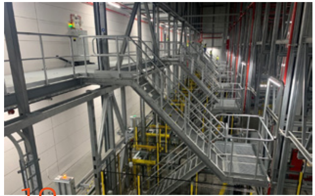
18 Highbay Warehouse Terneuzen
